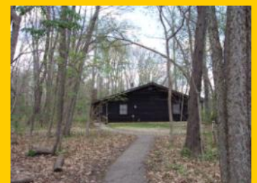
South Side of Lodge
